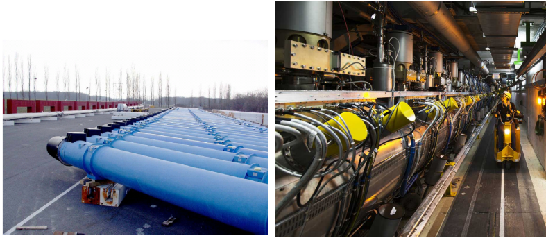
Figure 17.8: Left: LHC dipoles waiting for installation. They are 15 m long, weigh 35 tons, maintain up to B = 8 T magnetic field at T = 1.9 K. Right: The radio-frequency cavities accelerating the particles in the LHC ring
